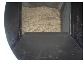
8: Picture looking down the pedestal [with flash on] showing the short urine separating plate and the soak in the bottom of the vault.
