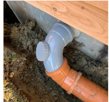
3: The grey pre-assembled urine outlet in place
