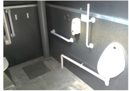
Urinal fitting and grab rails.
