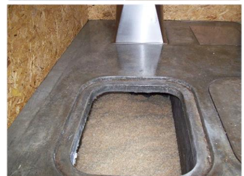
Use pedestal fix down (B4) at rear. The floor was supplied waxed
