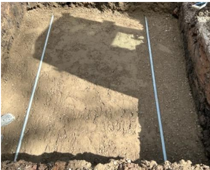
1: The excavation and the concrete screed levelled off.
