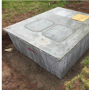
2: Showing concrete around the vaults.
