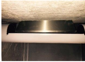
9a,9b: One into the active vault showing the rake in place and one showing the bottom of the stainless-steel urine separating plate over the urine collecting gutter.
