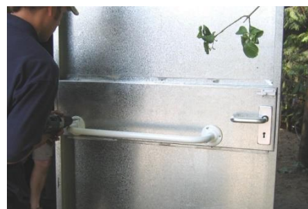
Grab rail being attached to the door.
