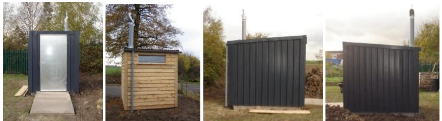
5a,5b,5c,5d: One of each elevation of the building from outside including the full height of vent pipe on at least one elevation. Corner and roof flashings should be in place.
